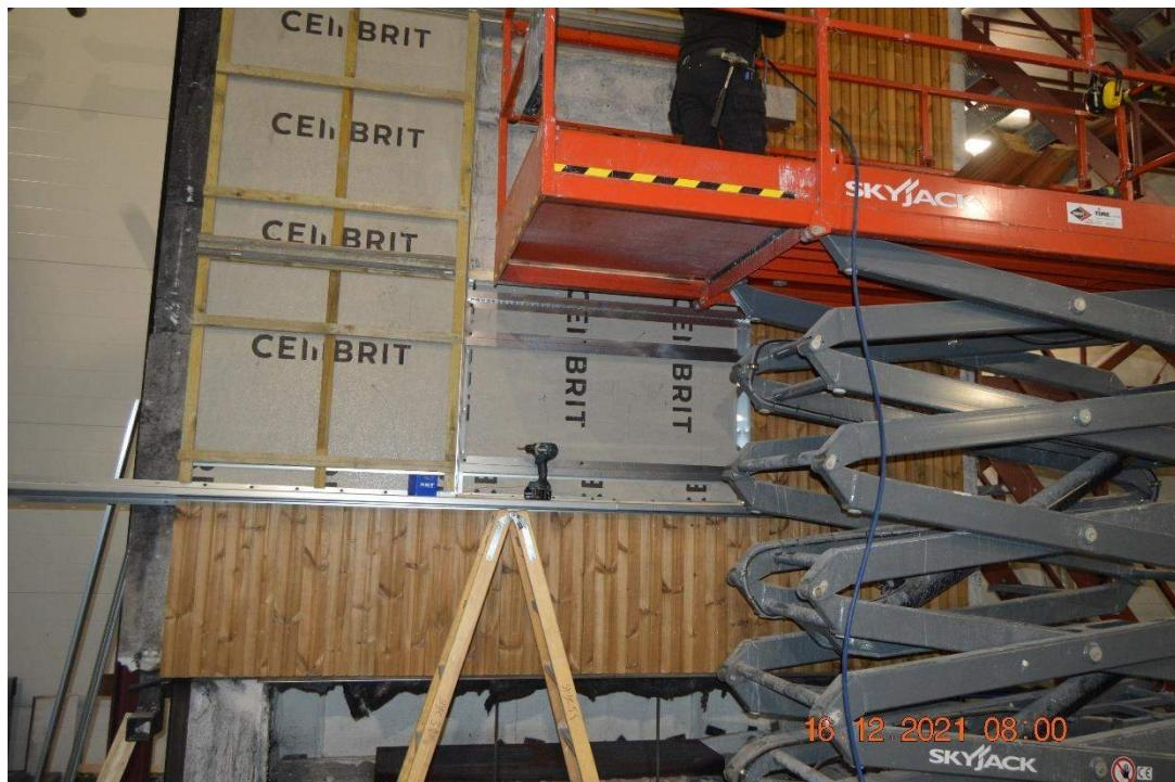
Photo No. 7 Cladding being mounted
