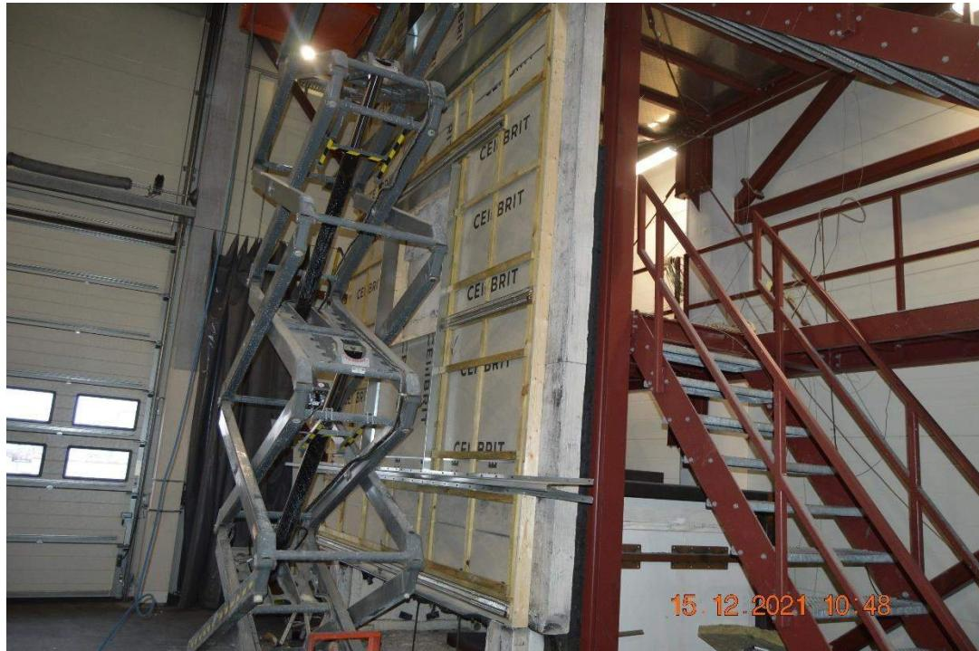
Photo No. 5 Battens, fire stop and horizontal fire screens during mounting
